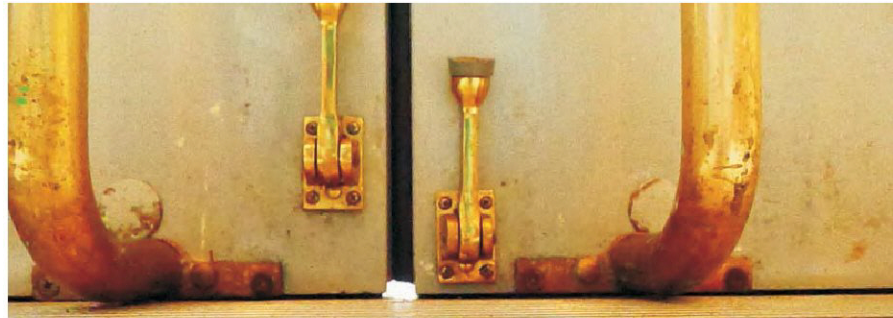
A mouse's eye view of the space between two double doors. Mice enter between these two very strong steel doors at will via the chewed out rubber gasket
